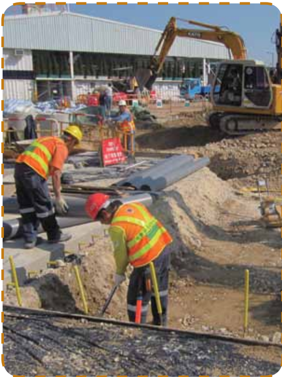
隧道進口斜路建造工程 Construction of approach ramp
