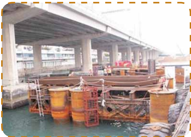
鑽孔樁工作平台建造工程 Construction of Bored Pile Working Platform
