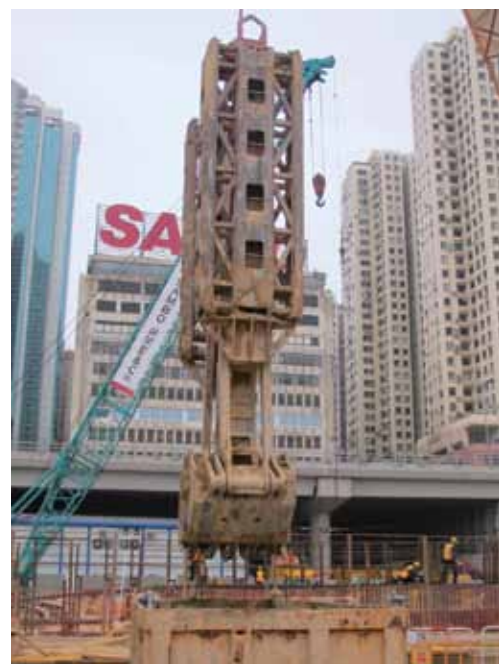
重13公噸的抓斗 Grab in weight of 13 tonnes
