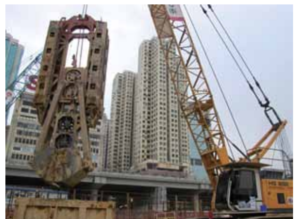
機械式挖土抓斗 Mechanical Excavation Grab
